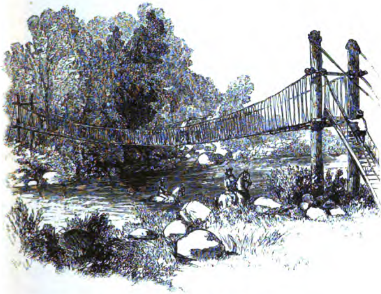
COWHIDE BRIDGE OVER THE RIMAC.
